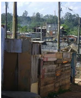
Figure 3a – house that was considered very poor
